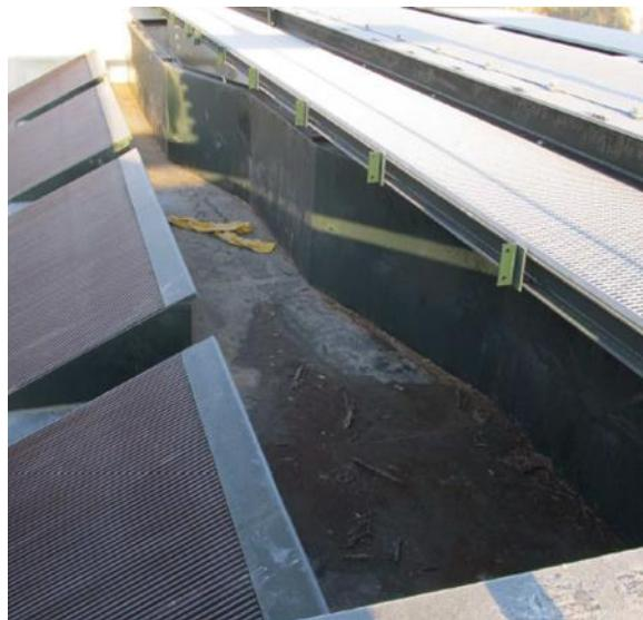
**Figure 26.** Chute at the top of an inclined bar rack. The outflow goes from the top to the bottom in the photo and the chute expands as the downstream migration outfalls run into it (photo D. Courret - OFB).
