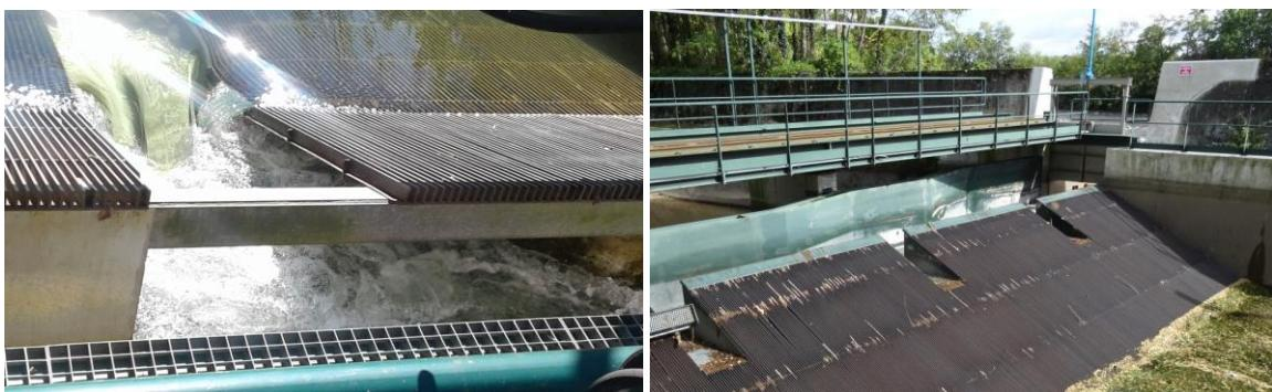
**Figure 24.** Outfalls at the top of the inclined bar racks (photos P. Sagnes – OFB).
