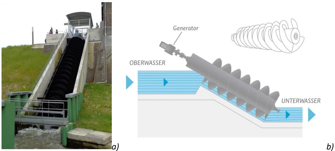
**Figure 5.** a) "Hydrodynamic screw-type turbine (photo P. Sagnes – OFB); b) operating principle ([www.landeskraftwerke.bayern](http://www.landeskraftwerke.bayern)).
