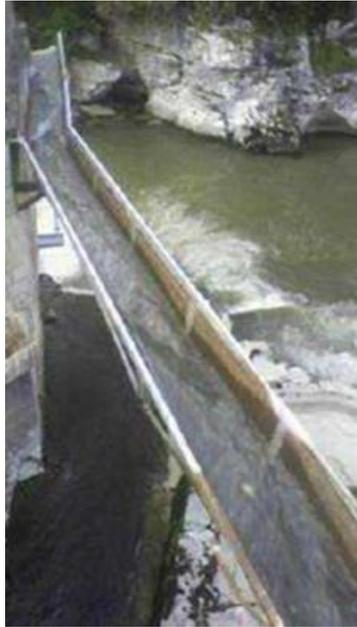
**Figure 27.** Transfer system of the downstream migrating fish, downstream of a bar rack and a collective chute (photo D. Courret - OFB).
