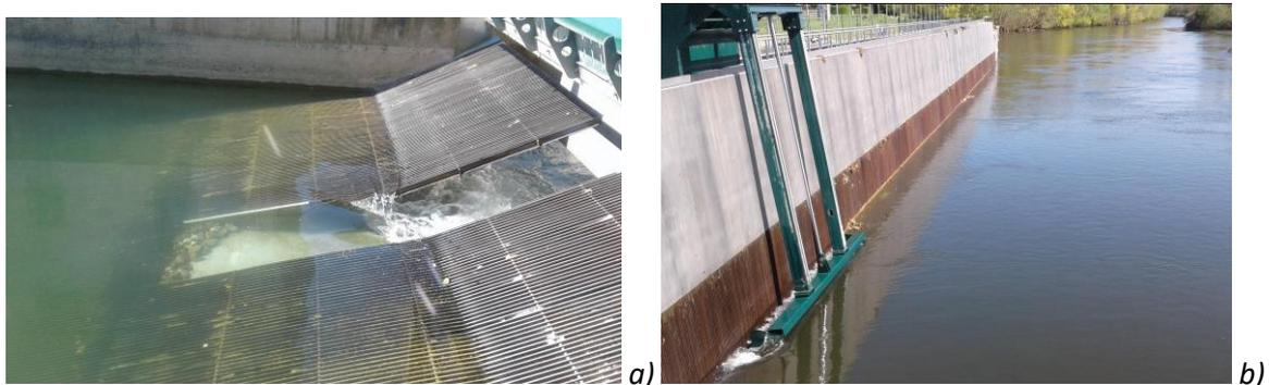
**Figure 6.** Fish-friendly water intakes. a) inclined bar rack; b) Angled bar rack (photos P. Sagnes - OFB).
