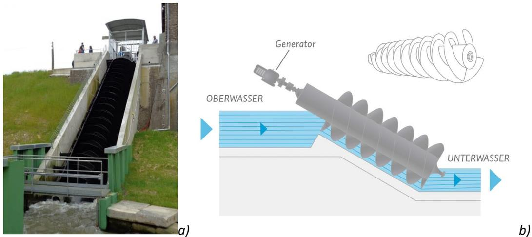
**Figure 5.** a) "Hydrodynamic screw-type turbine (photo P. Sagnes – OFB); b) operating principle (www.landeskraftwerke.bayern).
